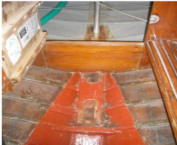
View of Horn Timber From Inside
